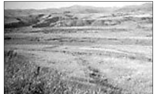
Scar caused by the NGP pipeline.
