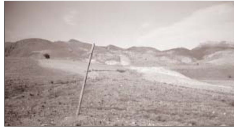
Scar left by the East Anatolian Natural Gas Pipeline (NGP) near Erzurum, north-eastern Turkey. The BTC pipeline would run alongside the NGP for 40% of its length in Turkey, between Erzurum and Sivas. (Greg Muttitt, PLATFORM)
